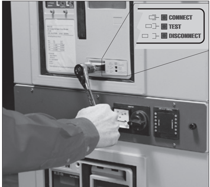
Figure 12. Levering Position Indication
